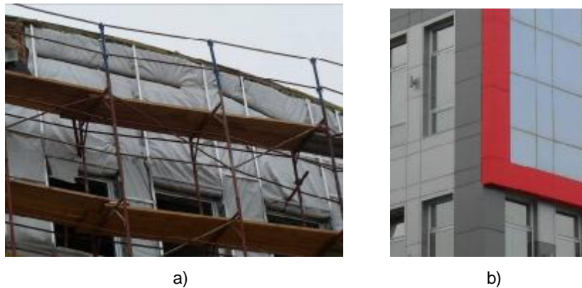
Slika 2. a) Nepravilno postavljena vodozaptivna folija; b) Detalj strukturne fasade prekriven pločama alukobonda, s visokim prozorima i zid-zavesom Figure 2. a) Badly placed waterproof sheeting; b) A detail of structural facade covered by alubond plates, with high window and wall curtain
